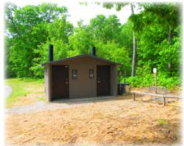
Restrooms (Hadicap Accessible)
